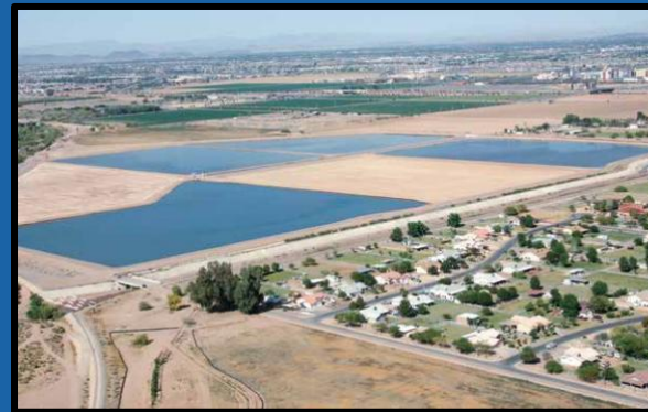
New River-Agua Fria River Underground Storage Project (NAUSP)
